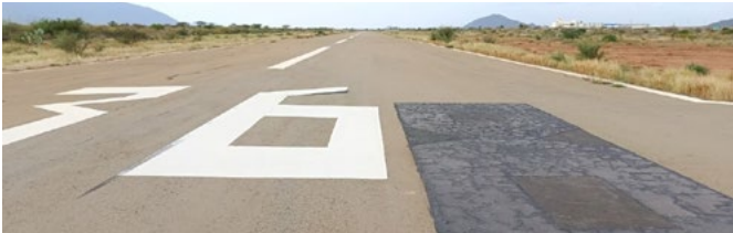
Ongoing construction of the Ikanga Airstrip in Voi constituency. Upon completion, the facility will enhance regional connectivity, boost tourism, and strengthen emergency response capacity.
